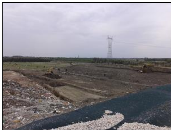
Figura 1: area in scarifica (01.10.2015)
